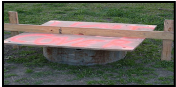
Example 2: Labeled Hole Cover 48"x48" 3/4" plywood with 2x4 secured across the top and held in place by two 2x4 stakes.
