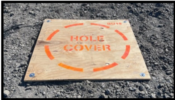
Example 1: Labeled Hole Cover 48"x48" 3/4" plywood secured with 12" anchor spikes and washers.
