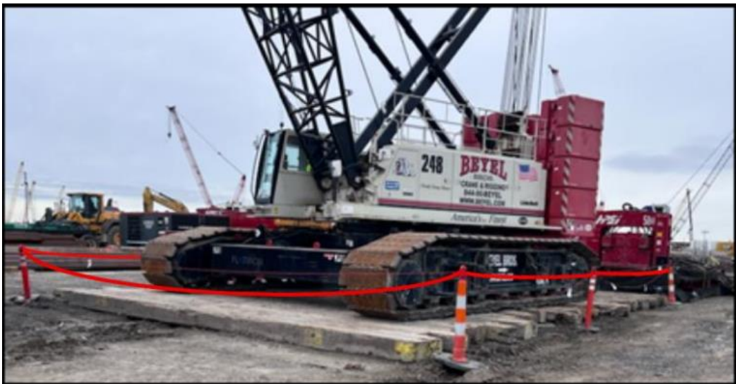
Example 2: Perimeter of Crane Barricade
