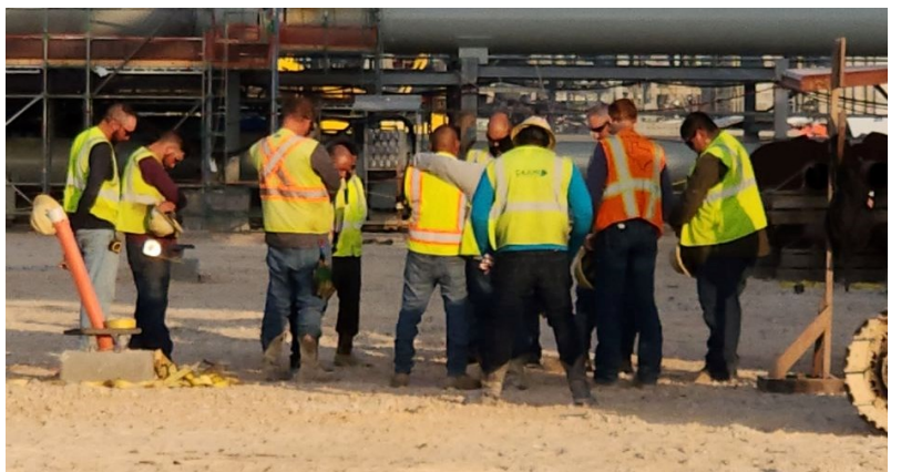
Crew praying before beginning work
